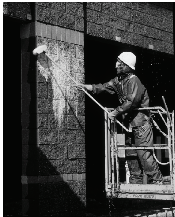
Figure 1—Pressure Chemical Cleaning (photo courtesy of PROSOCO, Inc.)
